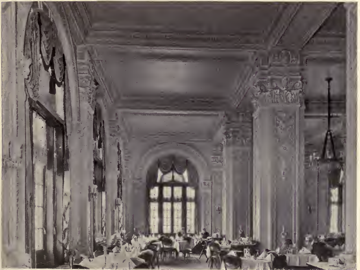
DINING ROOM, LOOKING EAST HOTEL WEBSTER, CHICAGO, ILL. FRIDSTEIN & CO., ENGINEERS
